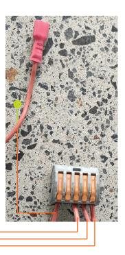
Connect One of the Live wirng of each heating elements and one wiring from 3. Step 2 to a 5-way cage clamp connector. Repect the same to another 5-way cage clamp connector.
