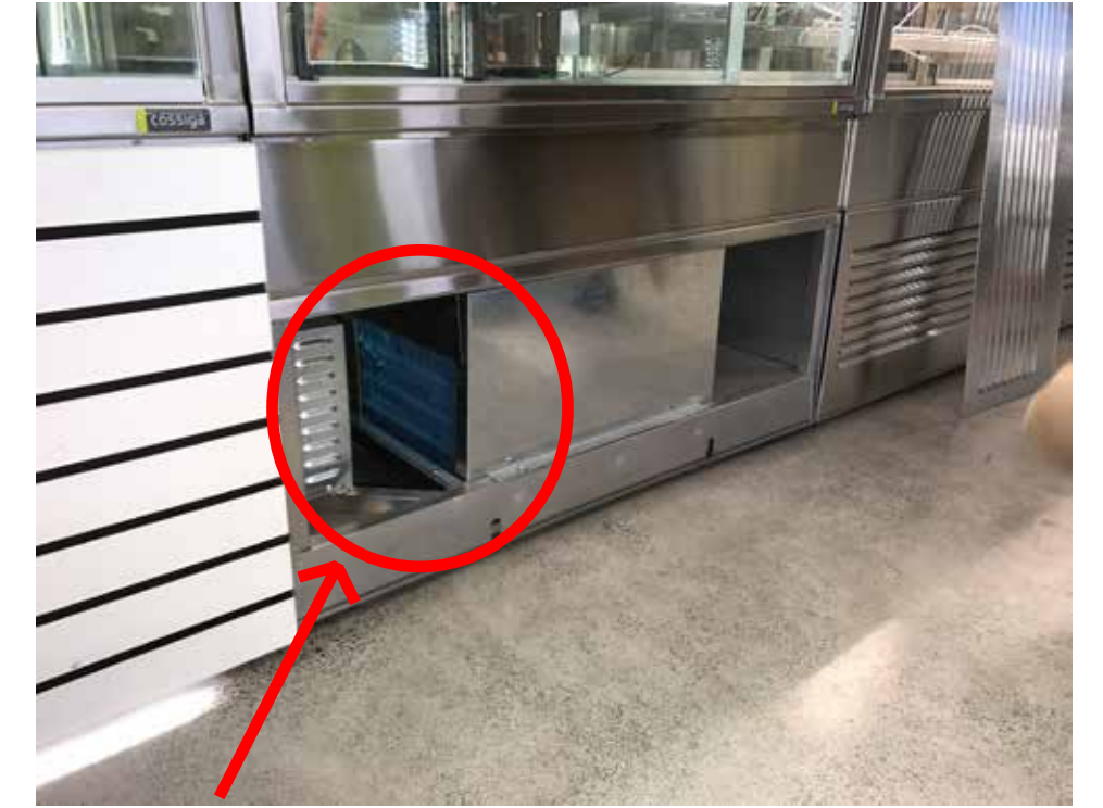
Remove Grill to access condenser
