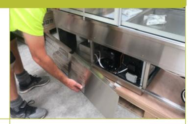
2. Unscrew and remove the front panel
